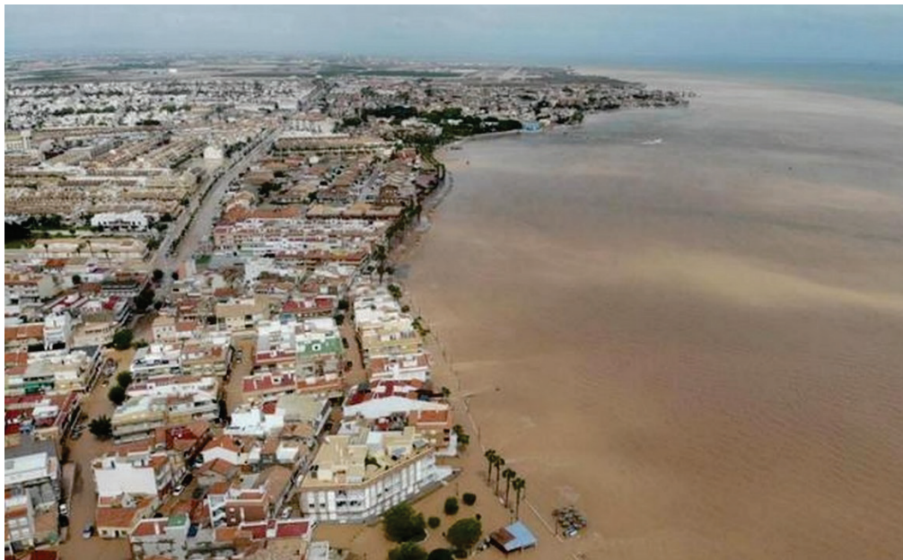
Figure 5. Aerial view of the effects of DANA on Los Alcázares and the Mar Menor. Source: La Verdad, 14th Sept 2019.
