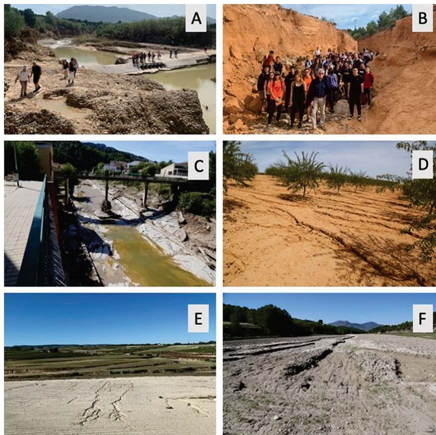
Figure 1. Views of the impact of the DANA of 12 September 2019 at the study area of river Canyoles watershed. View of the river Canyoles talweg after the flood in Granja de la Costera, (A), gully formed as a consequence of the mismanagement of the railway flows at Font de la Figuera (B), talweg of the river Canyoles in Moixent with the removal of the sediments (C), almond plantation affected by rilling in Font de la Figuera (D), rill development in sunflower fields in Moixent (E), and barley field after tillage with wide gullies in Font de la Figuera (F).
