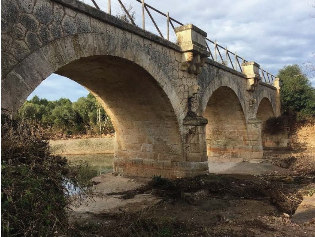
Figure 7. Rail-road bridge over torrent de ca n' Amer, with a total span of 100 m 2 . During the flood in 2018 it worked to its limit, being used as flow control point.
