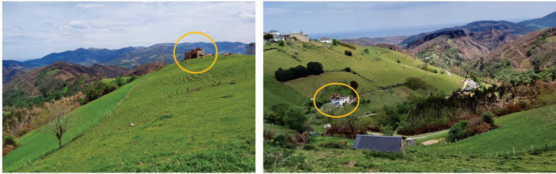
Figure 3. Buildings with a low risk of direct exposure to forest fire but damaged by the arrival of burning embers from nearby pine plantations (indirect exposure) during the Foyedo forest fire. Locality of Lago (council of Valdés, Principality of Asturias, Spain).
